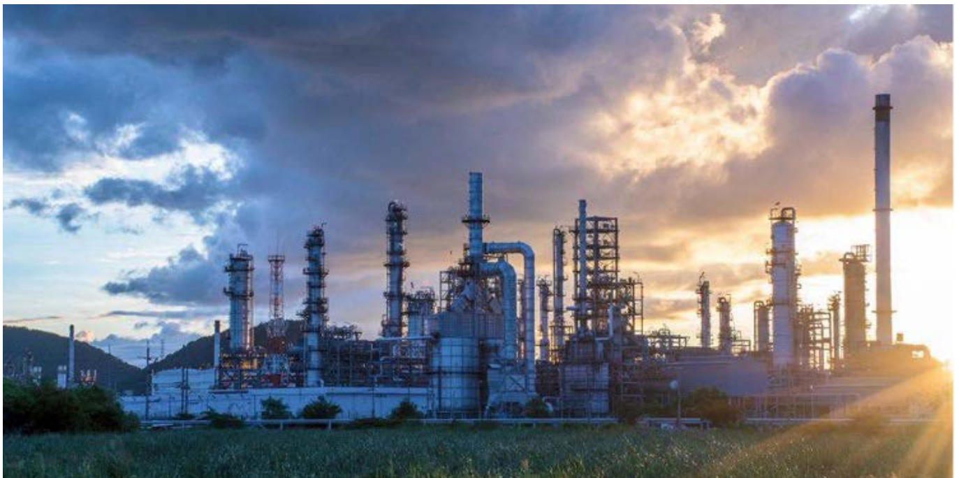
Figure 1: A Steam Methane Reforming Unit
